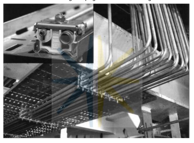
The ETIN Tubing Clamp is patented. Manufactured by Øglaend System of Norway.
