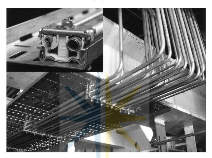
The ETIN Tubing Clamp is patented.
